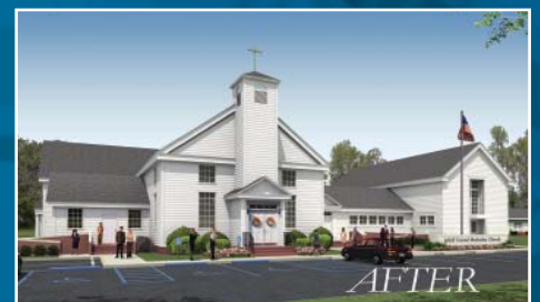
JOLLIFF UNITED METHODIST CHURCH CURRENTLY UNDER CONSTRUCTION
